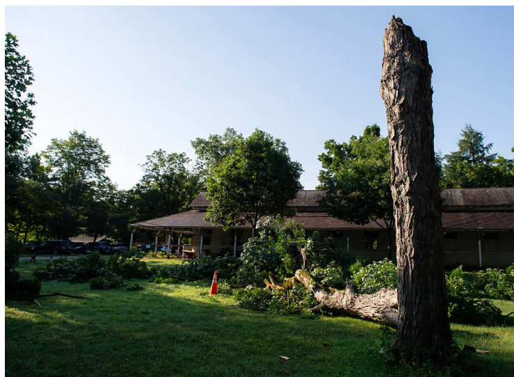
Storm damage at Saratoga | Sarah Andrew
