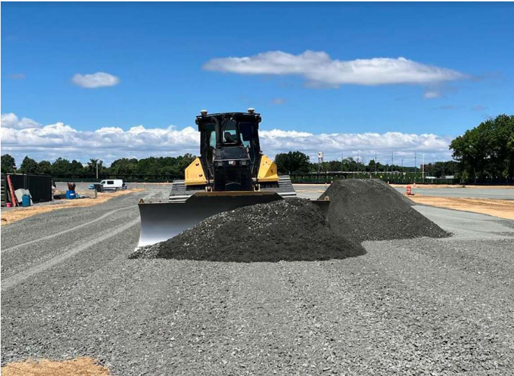
Construction of Tapeta surface at Belmont Park
