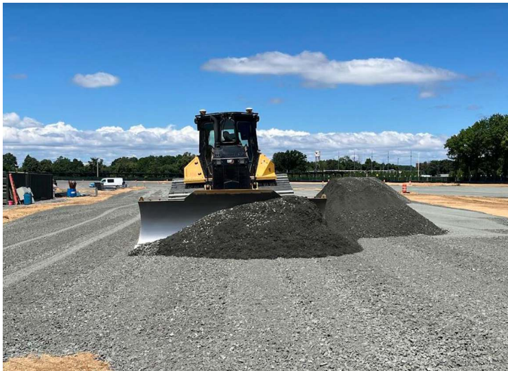
Construction of Tapeta surface at Belmont Park
