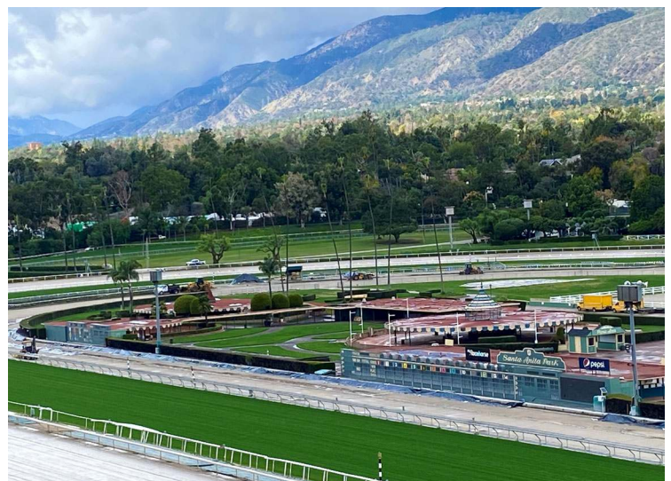
Santa Anita construction of new Tapeta track | Santa Anita
